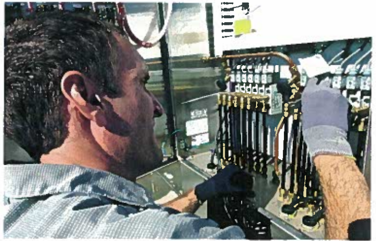
Trey Cain manually operates air valves on the tertiary filters at the Lincoln plant.
