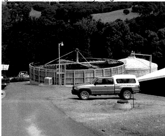
Trickling Filter at San Andreas Wastewater Treatment Plant
